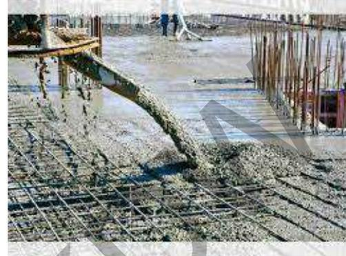
MENGGUNAKAN PLAT LANTAI DENGAN BAHAN BETON KONVENSIONAL DENGAN KETEBALAN 15-20 CM.
